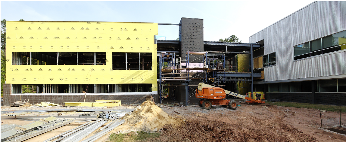
The building addition as of June 25, 2008
